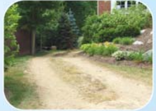
Without GEORUNNER® System: Typical rutting and turf damage
